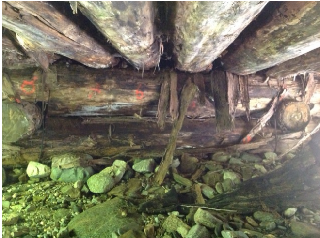
Right Bank Abutment when facing downstream
