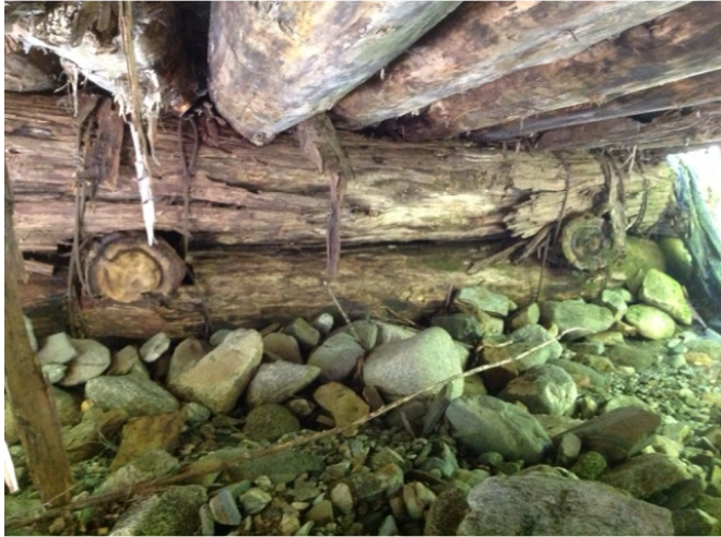
Left Bank Abutment when facing downstream
